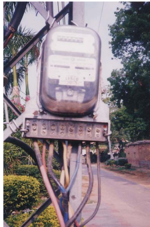
Meter without box & terminal cover
