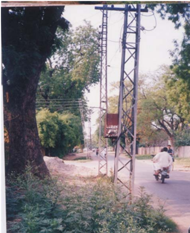
Poles out of alignment
