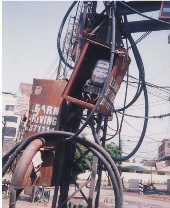
Meter hanging with support of cotton cord
