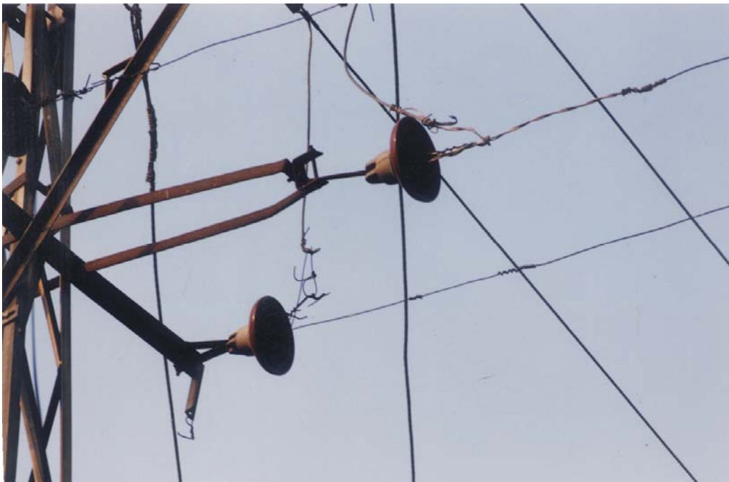
Jumpering interconnection of 11kV line from Main to Sub-main
