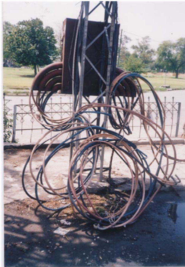
Extra Length of live cable retained and lying along heavy traffic road
